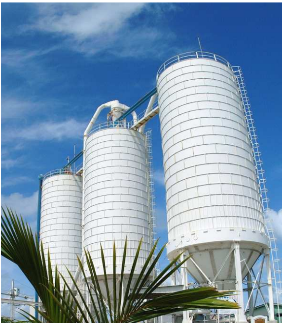
Lafarge Maldives Cement Plant
